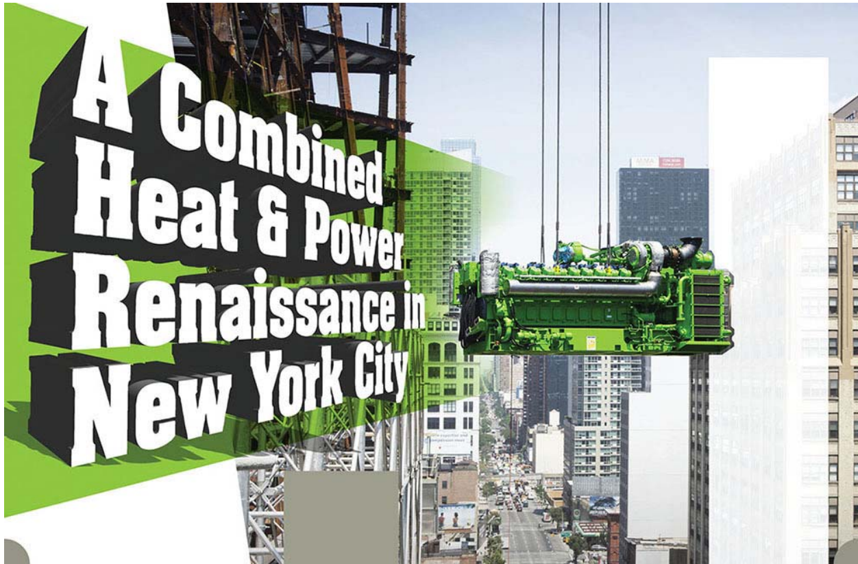
One of four Jenbacher J620 gas engines being lifted by crane into place for the Hudson Yards project in New York City. Photo courtesy: GE
