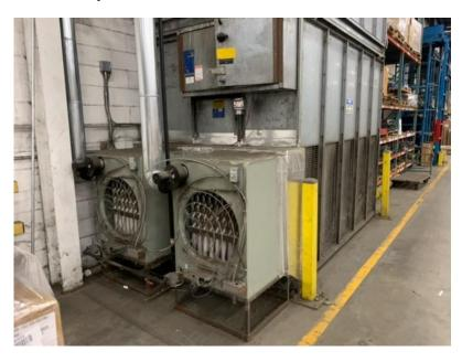
Someone had the bright idea to disconnect the flue pipe going through the wall and run the flue pipe inside to help heat the garage!
